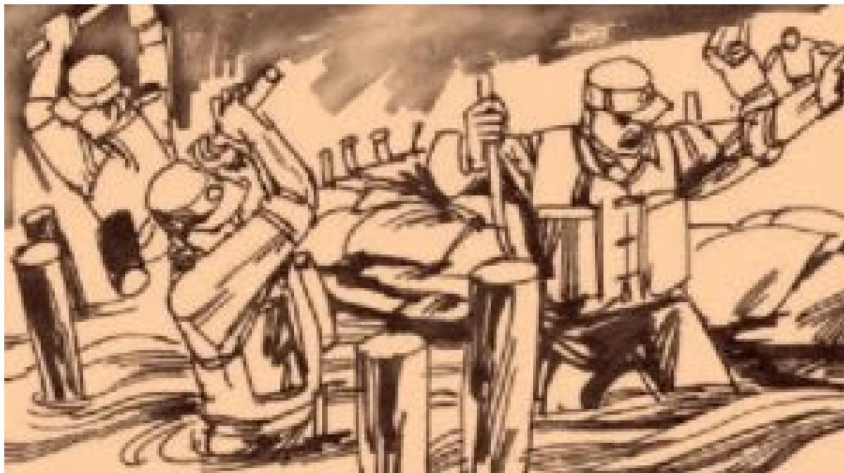
Later a 200-member special force group from Zhangjiakou, who were trained in levee repair came, and build pilings around the rupture. Afterward, they used pilings to stabilize the prefabricated panels, then, they poured in mud and rocks, eventually sealing the opening.
